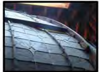
Before repair and restoration. ▶
